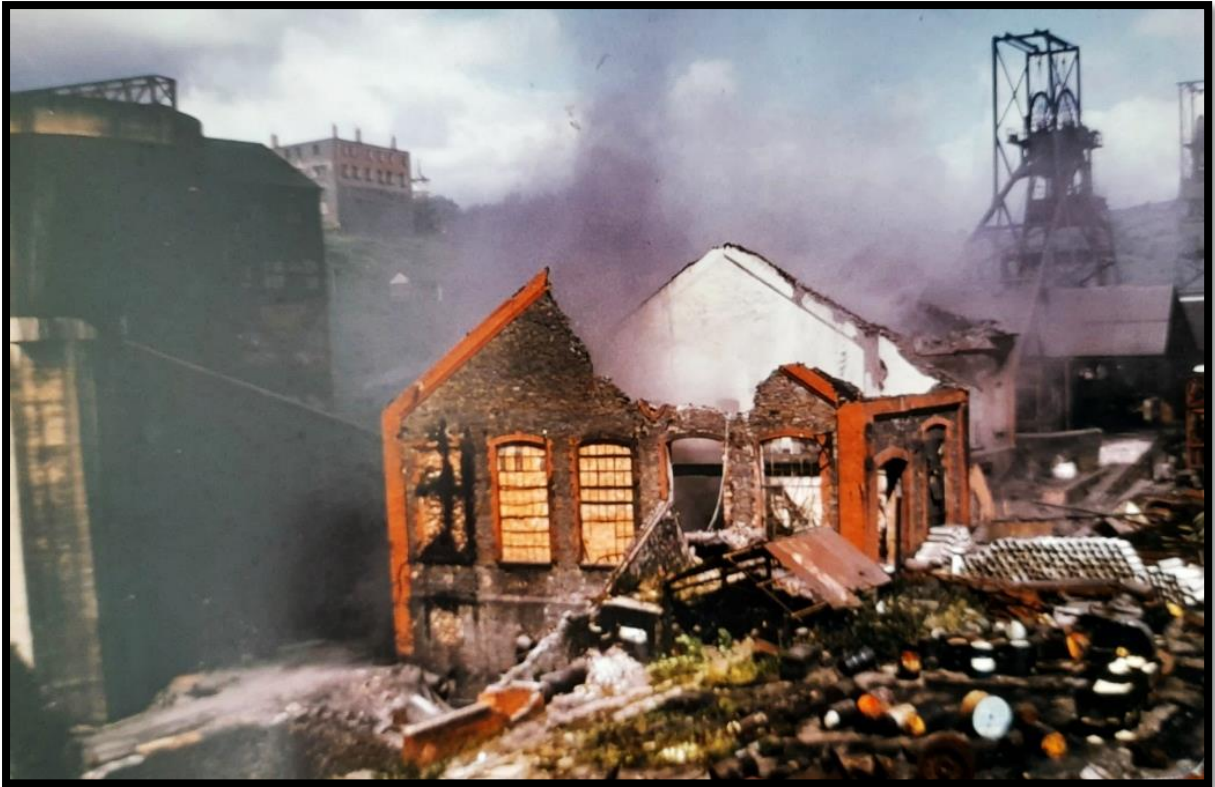
The demolition of Bargoed Colliery
