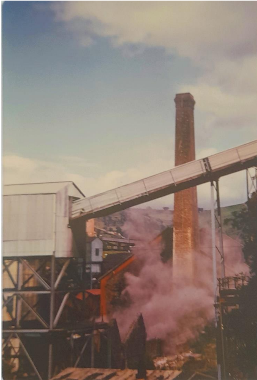
The demolition of Bargoed Colliery
